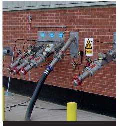
Pneumag installed at bulk material intake, ATEX rated.
